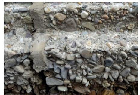
Figure 1: Concrete exposed to acid attack
