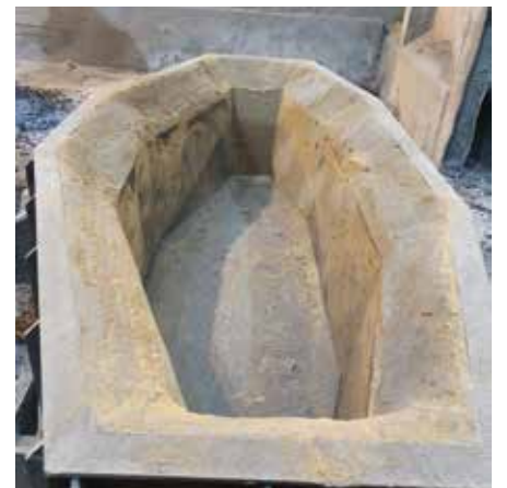
Figure 5: Tundish after lining with cement
