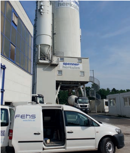
Figure 9: Demonstrator test at ready-mix concrete plant of Spenner Herkules GmbH
